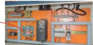
'All in One PLC card' for Mechanical Loom
